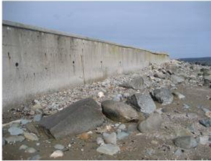
Fig. A-18. Mass concrete seawall
