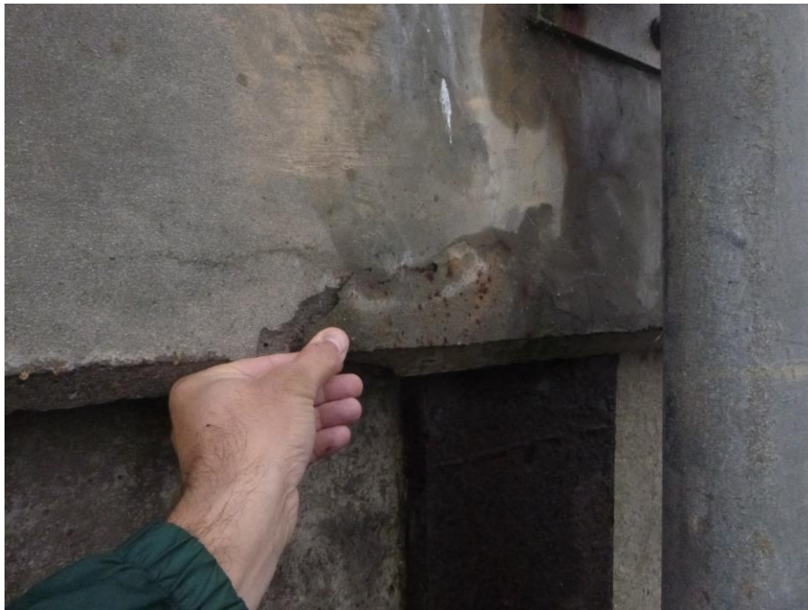
3(b). Repairs for cracks on pile cap face
