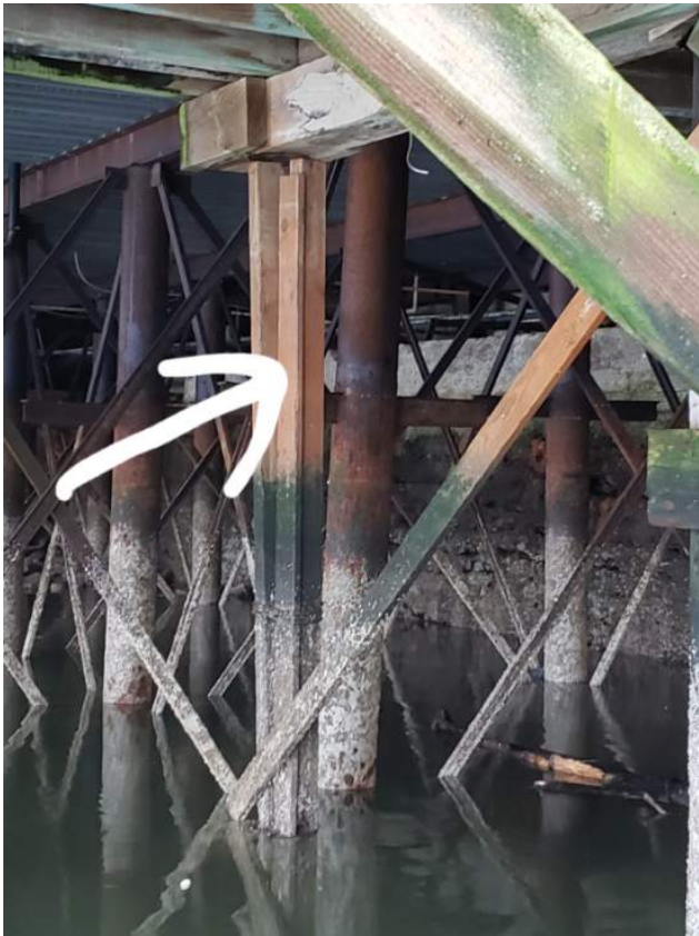
Figure 1 A bundle of pressure treated lumber in the place where a piling should go; base has shifted, lumber is not in contact with beam.
