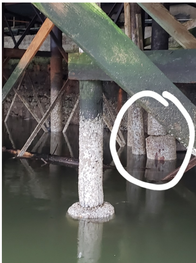
Figure 1 A bundle of pressure treated lumber in the place where a piling should go; base has shifted, lumber is not in contact with beam.
