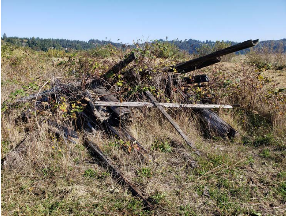
Figure 4 Old Wooden Pilings on Hall Property
