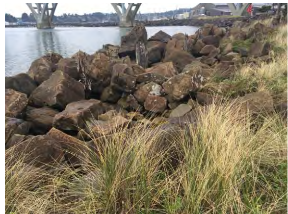
Picture #48. Rock shoring
