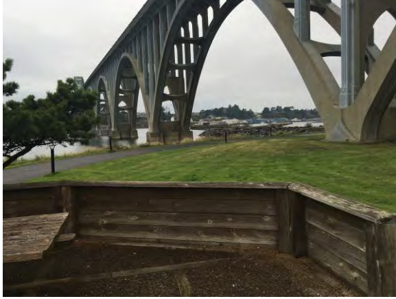
Picture #31. Yaquina Bay bridge
