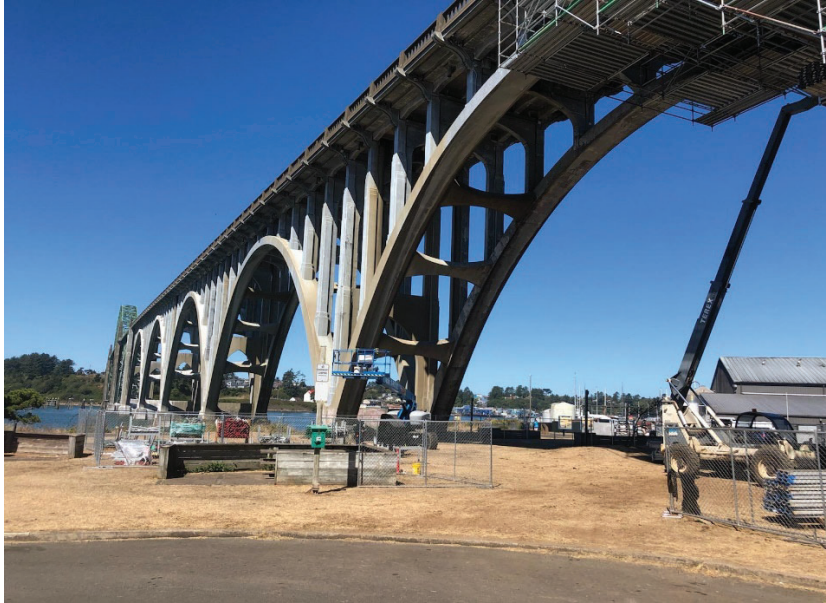
Yaquina Bridge, Newport - ODOT Staging area – looking north
