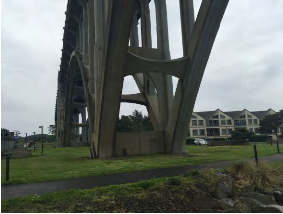
Picture #13. Bridge pier
