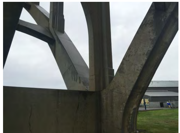
Picture #18. Bridge pier
