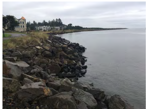
Picture #12. Rock shoring
