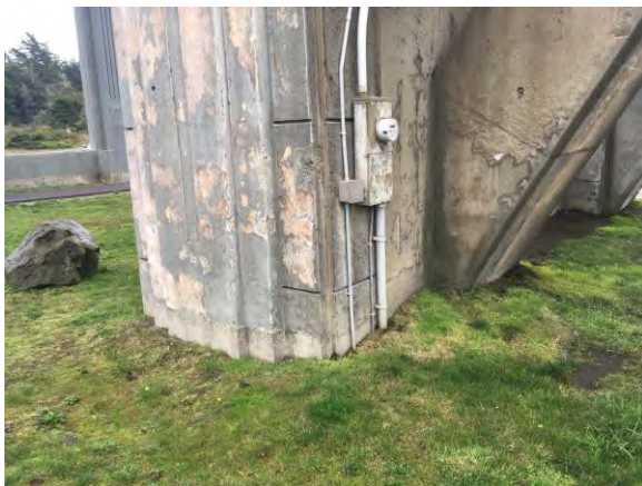
Picture #27. Bridge pier
