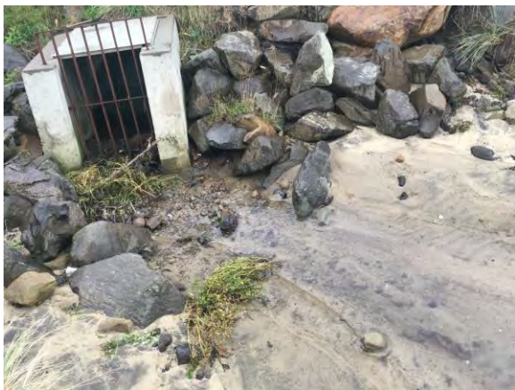
Picture #45. Drain outlet
