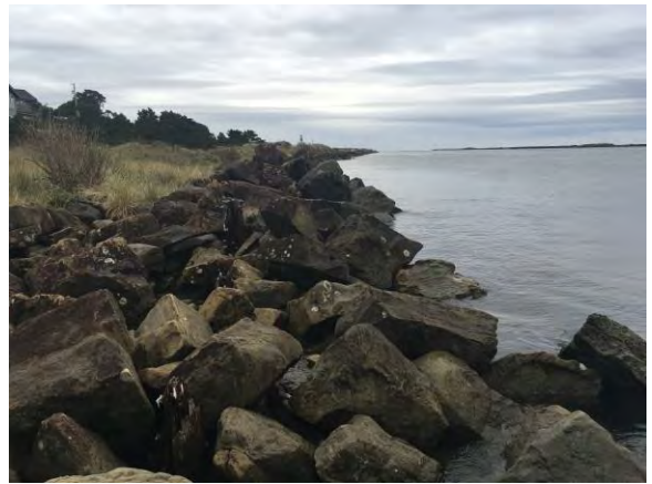
Picture #53. Rock shoring
