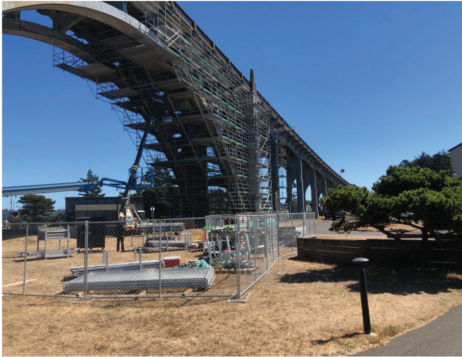
Yaquina Bridge, Newport - ODOT Staging area – Looking south
