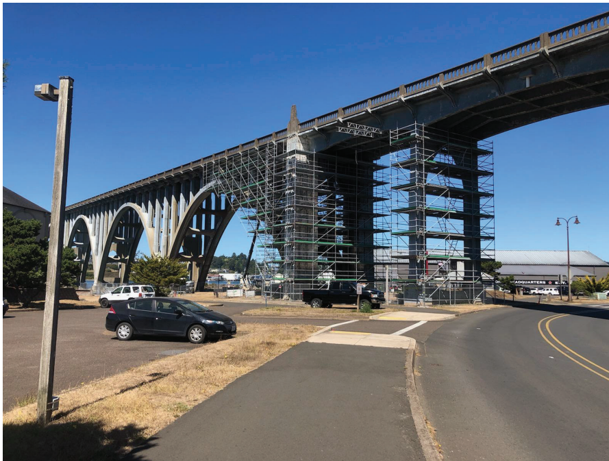
Yaquina Bridge, Newport - ODOT Scaffolding looking northeast
