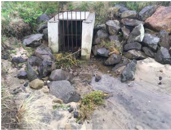
Picture #44. Drain outlet
