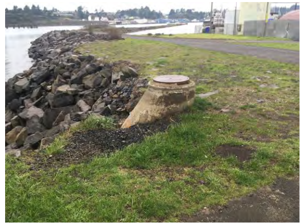
Picture #11. Sanitary sewer manhole
