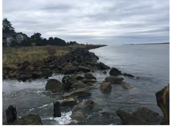
Picture #52. Rock shoring
