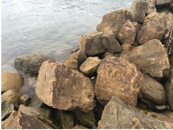
Picture #49. Rock shoring
