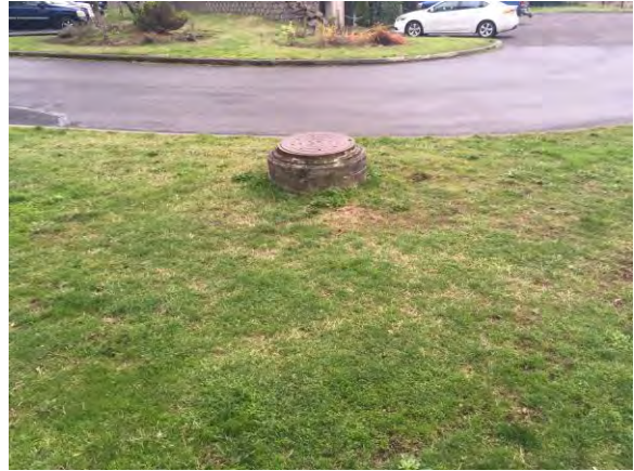
Picture #22. Sanitary sewer manhole
