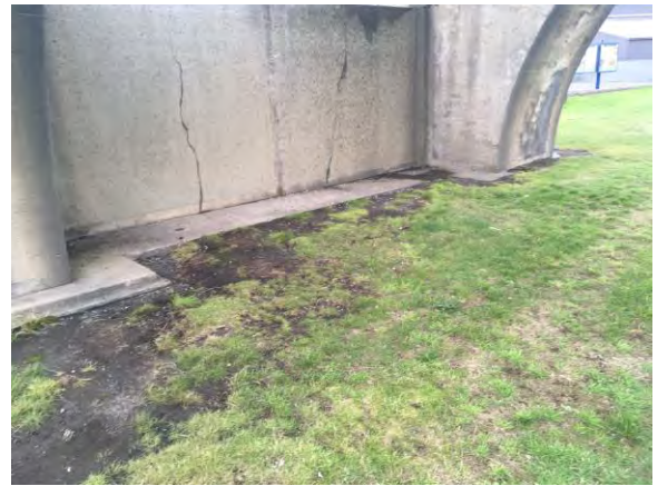
Picture #17. Bridge pier
