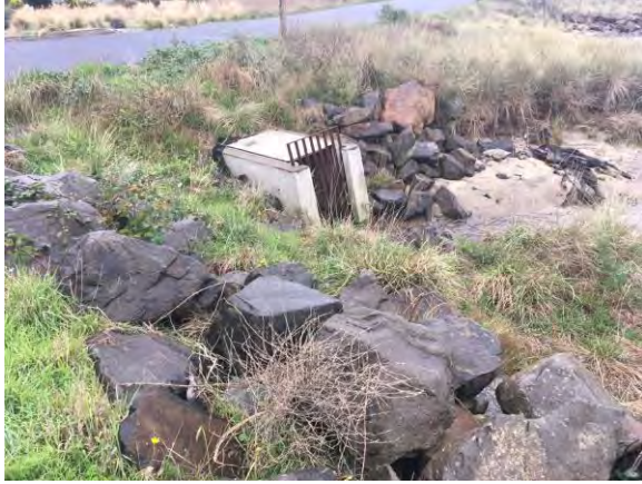
Picture #43. Drain outlet
