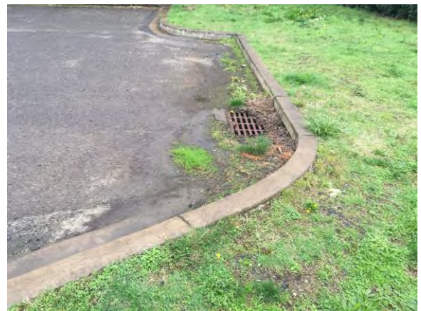
Picture #36. Drain in parking area
