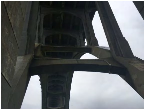
Picture #26. Bridge pier
