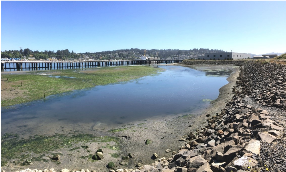
Top photo (A): Taken from top of bank at west end of Area A, looking to northeast.
